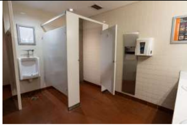
Men's Rice Lobby bathroom
