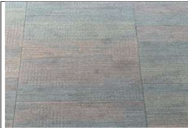
There is low pile tile carpet flooring on the third floor of the Shoctor Lobby.
